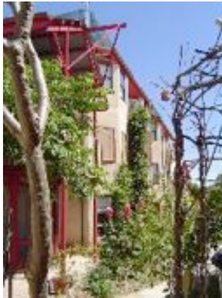
Christie Walk in central Adelaide - 27 green low-energy households on a mere 2000 m 2 http://www.urbanecology.org.au/christiewalk/
