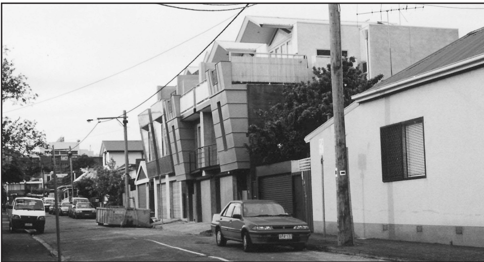
The future according to Melbourne 2030 — huge multi-storey boundary-to-boundary developments with little or no ground level open space, lots of balconies and plenty of overlooking!
